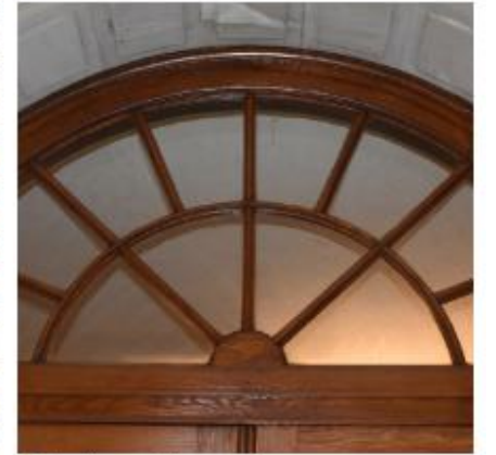
Stained wood doors and transoms.
