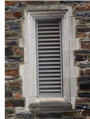
Louvered window replacement.
