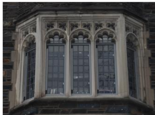
Bay window configuration with ornate limestone tracery.
